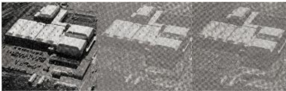
AN EXACT duplicate of the NBC color studios recently completed at Burbank, Calif. (l), will be constructed there. Another major color studio will be built in Brooklyn, adjacent to the existing NBC studio.
